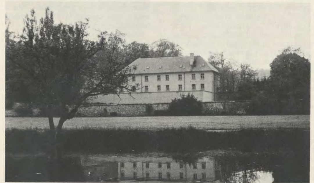
Rear view of Dosnon, the Catering School in Couvrelles, near Paris.
