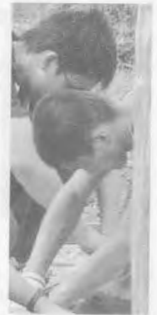
Preparing the floor and the posts for the roof of the new facility at the Holy Infant Orphanage.
